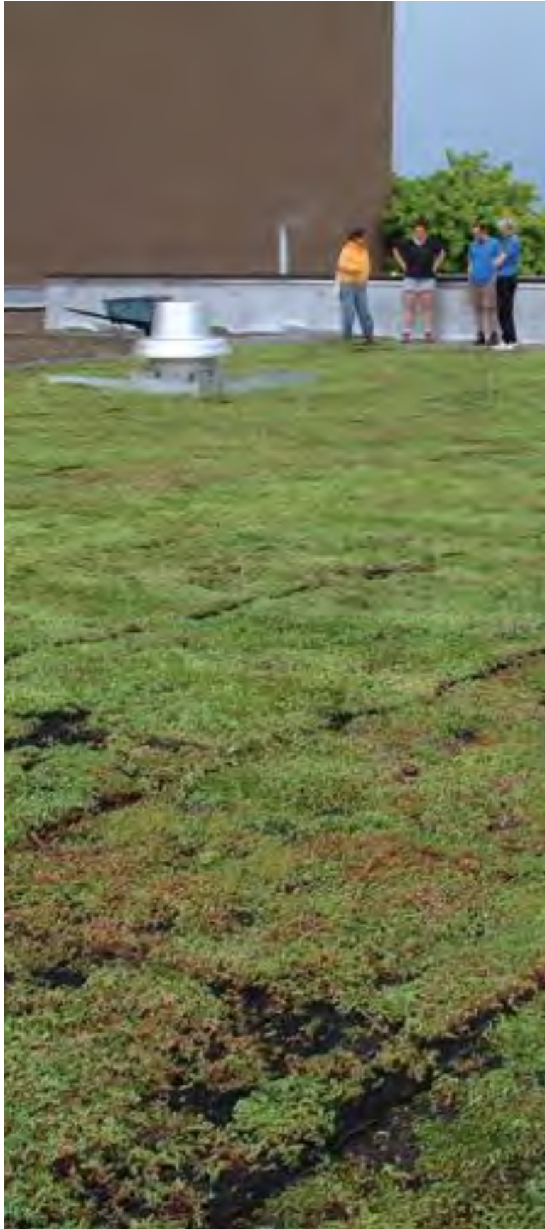
Green roofs reduce the heat island effect, retain water, provide insulation and promote evapotranspiration.
