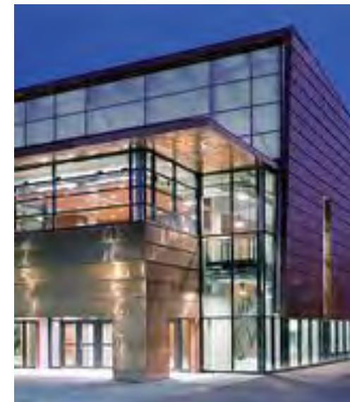
Copper cladding on this new building will patinate over time, providing a durable and attractive finish.
